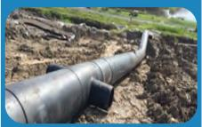
typical landfill leachate collection systems to protect the water and the environment from landfill contaminants. These systems use a series of high-density polyethylene riser shafts, which must additional have pipe continuously added to the riser as the landfill soil cover increases in height. The characteristics of HDPE pipe and fittings allow these systems to be continuously modified as the landfill progresses.
